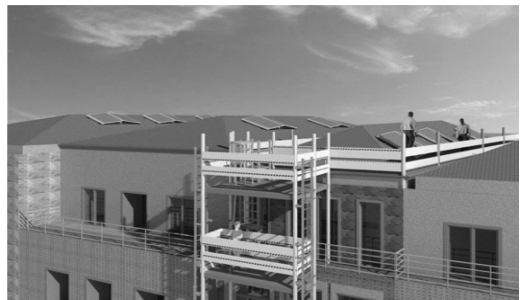
Figure 5. Positioning of workers during servicing of solar panels.
