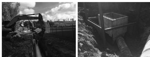
Figure 2. Construction of drainage networks for sewage and water supply.
