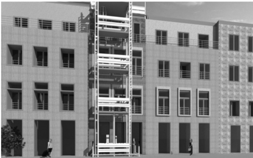
Figure 2. Placement of the scaffolds for façade works.
