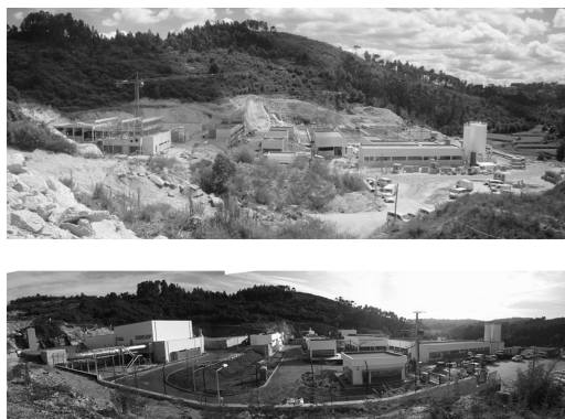
Figure 1. Construction of large sewage treatment plant.
