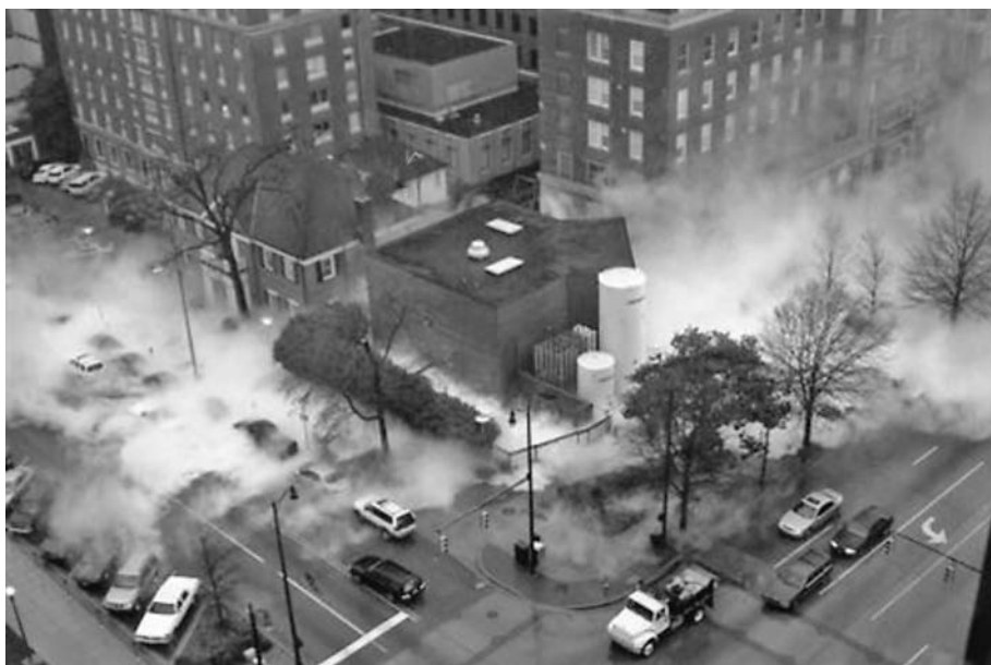
Figure 19.1. University of Alabama LOX spill. Eight thousand gallons of LOX escaped, making it temporarily impossible to assess either the primary tank or secondary reserve tank. Efficient implementation of predetermined protocol ensured that there was no adverse patient outcome despite peak use at the time of the incident. (Reproduced with permission from Schumacher SD, Brockwell RC, Andrews JJ, Ogles D. Bulk liquid oxygen supply failure. Anesthesiology 2004; 100:186–189.)
