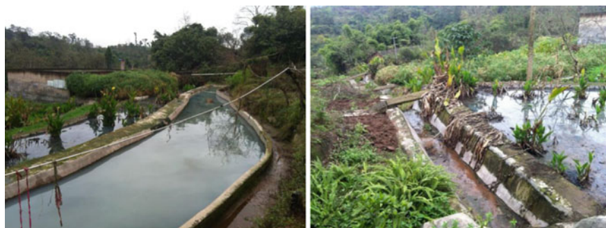
Fig. 10 Experimental ecological engineering with vegetation ponds and ditches for local water pollution treatment
