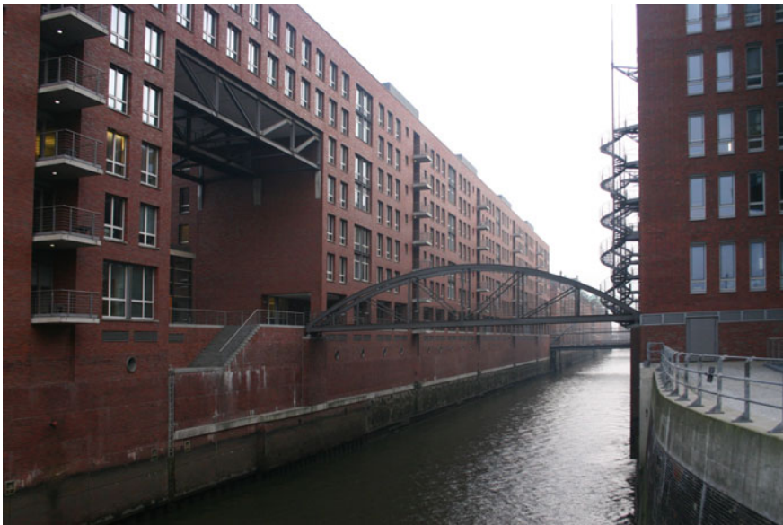
Fig. 7 A bridge in HafenCity, Hamburg that would allow connection between the buildings aboveground during flooding
