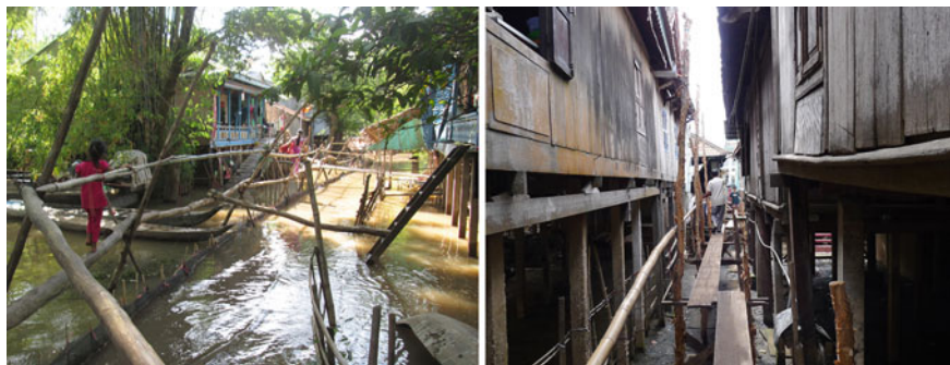
Fig. 5 Makeshift bridges in Vinh An (left; a monkey bridge) and Ha Bao (right) during the flood season
