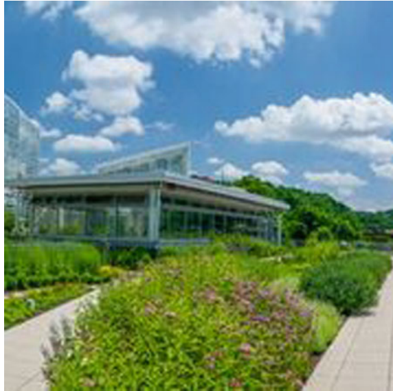
Fig. 7 Phipps' Center for Sustainable Landscapes highlighting green roof with tropical forest conservatory in background (Photograph by Paul G. Wiegman)
